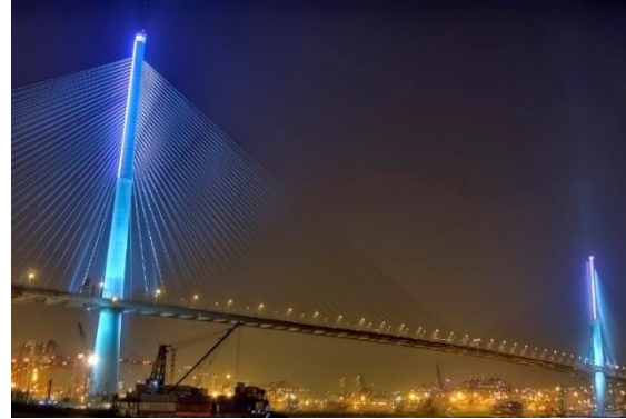
Bridge cables 橋梁鋼纜索
