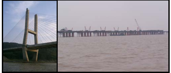
Fig. 8 Poyang Lake bridge and another bridge under construction nearby
