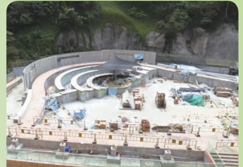
The Bricks Wall under construction
