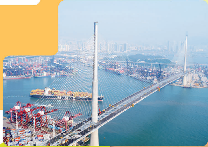
Stonecutters Bridge » (Courtesy of Highways Department)
