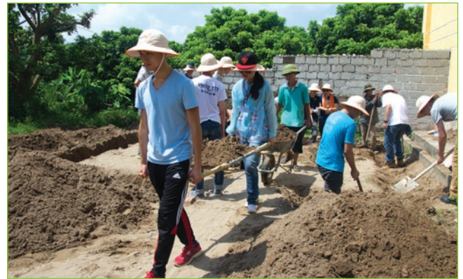
Students helped the local construction workers for ground excavation work
